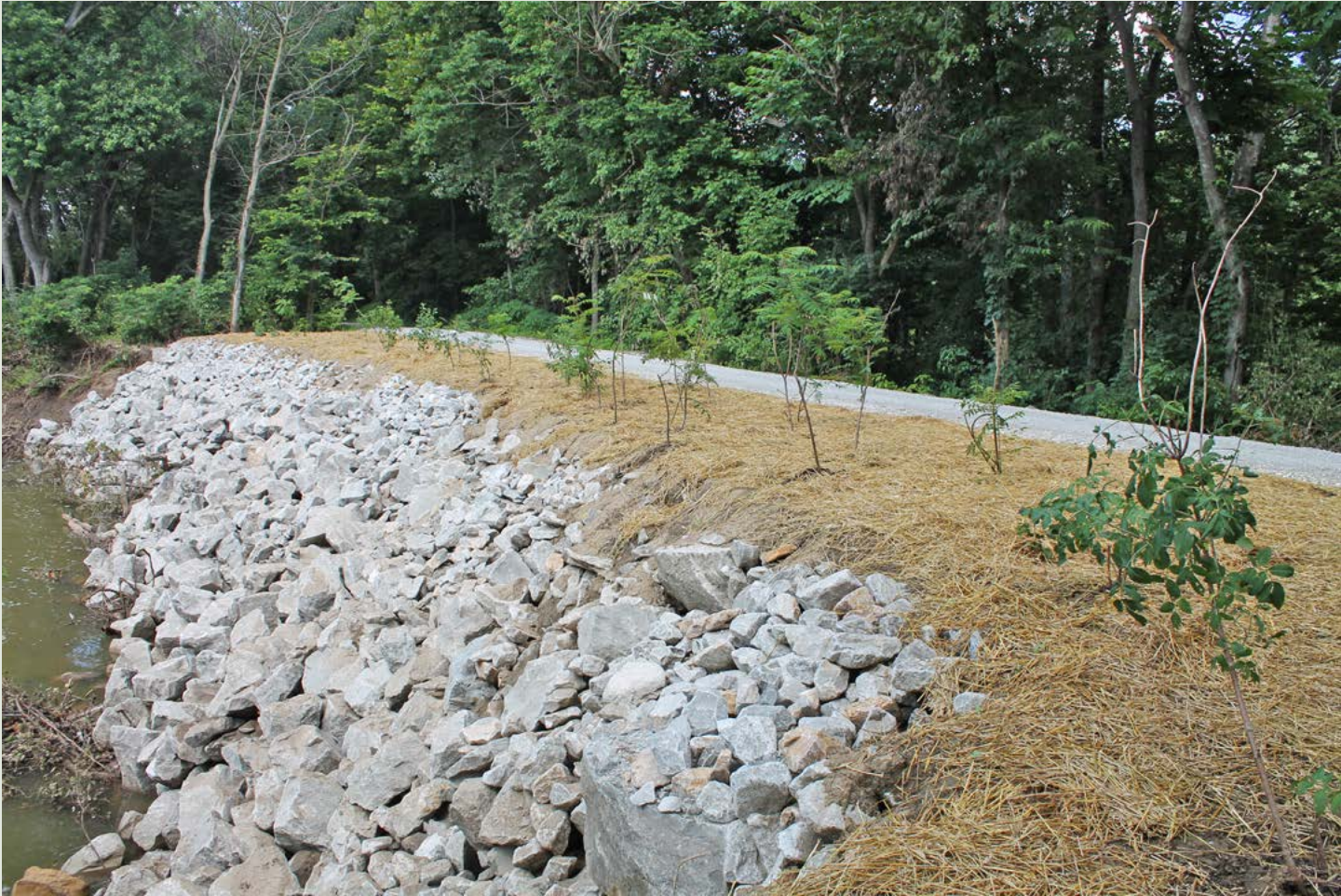
Streambed restoration on Hinkson Creek in Columbia, Missouri. The crest of the bank was seeded with river oats ( Chasmanthium latifolium ) and planted with stoloniferous (suckering) multi-stem native shrubs such as elderberry ( Sambucus canadensis ) and staghorn sumac ( Rhus typhina ) to quickly establish a network of anchoring roots. The creek has since been slowly depositing silt in the gaps among exposed boulders, which will allow Columbia to plant this rocky bank with sandbar willow cuttings this spring. Photo by Brett O’Brien
