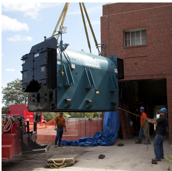
Workers position a new wood-fired boiler for installation in a municipal building in Curtis.
