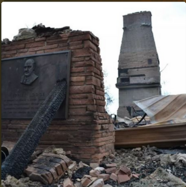
Ten cabins, Eppley Lodge, and the Scott Lookout Tower were destroyed in the fire (photo courtesy of Carson Vaughn).
