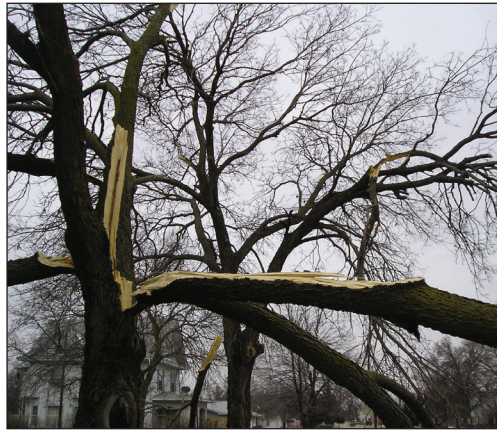
Trees with cracked or split trunks, water seepage or disturbed roots should be inspected by a professional arborist.
