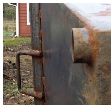
Handle and drain hole details of the Oregon Kiln.
